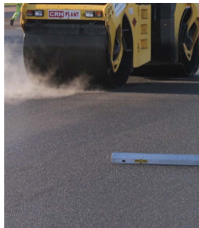
No RAP in Mix / Surface Regularity Testing
