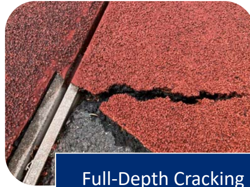
Improper Installation Depth
