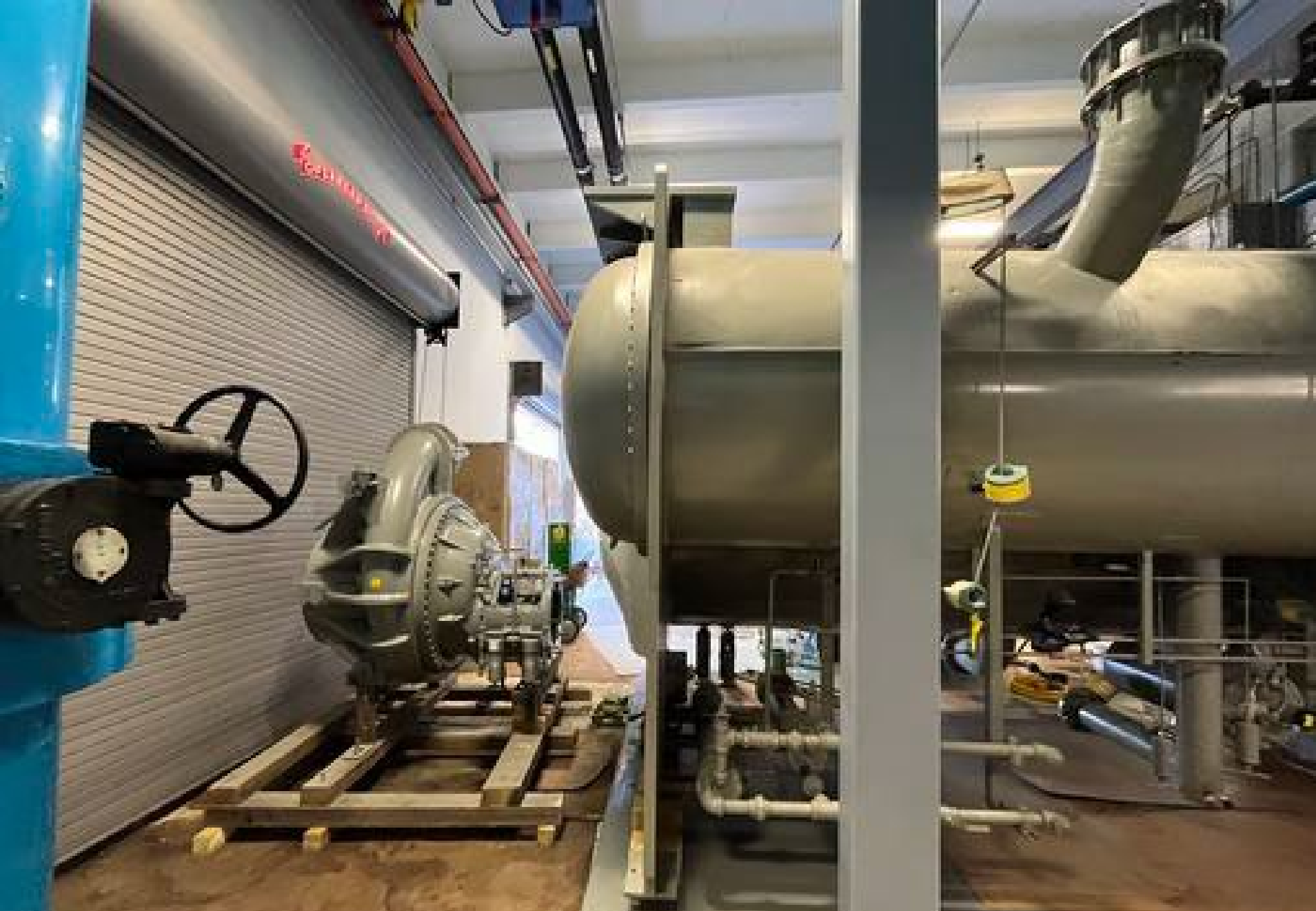
Building of Chiller # 5 Progress May 11, 2024
