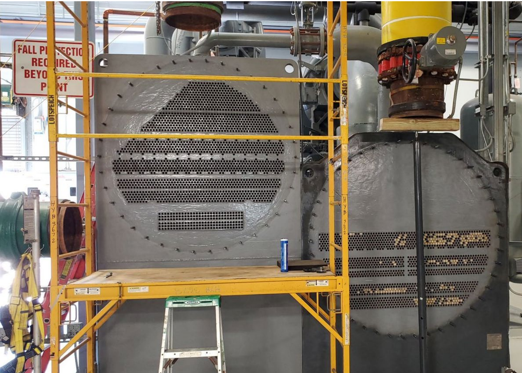
Chiller #2 Tube Sheets Following New Epoxy
