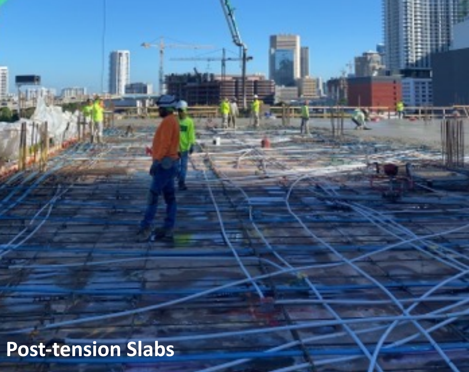
Integrated systems in slabs
