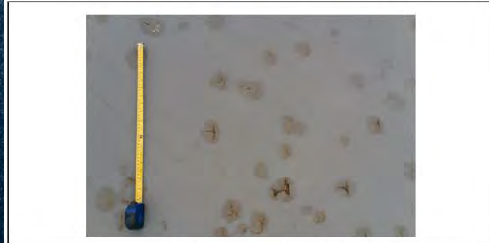
Fig. 3.1.1-2. Close-up of roof in Figure 3.1.1-1
