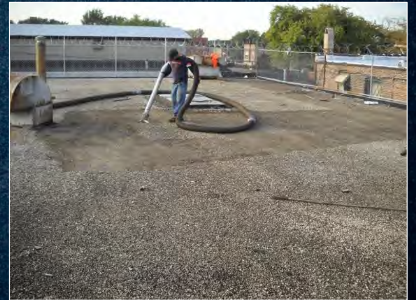
Wet Vacuum Gravel Removal
