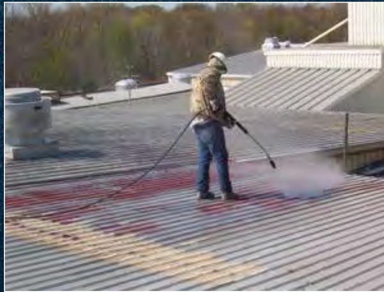
Pressure Wash/ Remove Loose Coating
