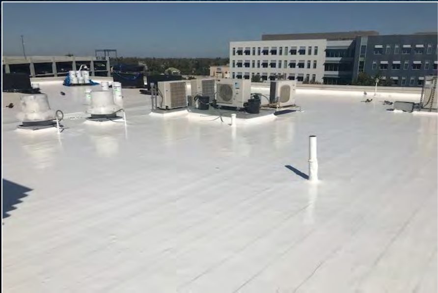
Modified Bitumen Roof Restoration
