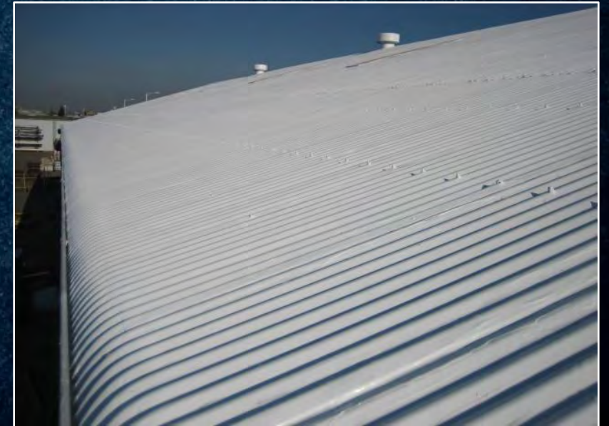
Metal Roof Restoration
