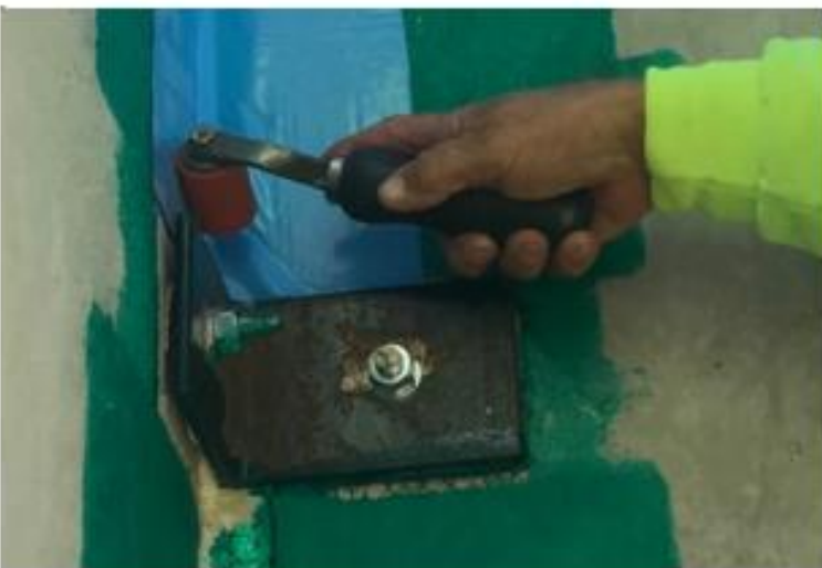
STEP 5: APPLY TRANSITION MEMBRANE AND ADHERE WITH WEIGHTED ROLLER
