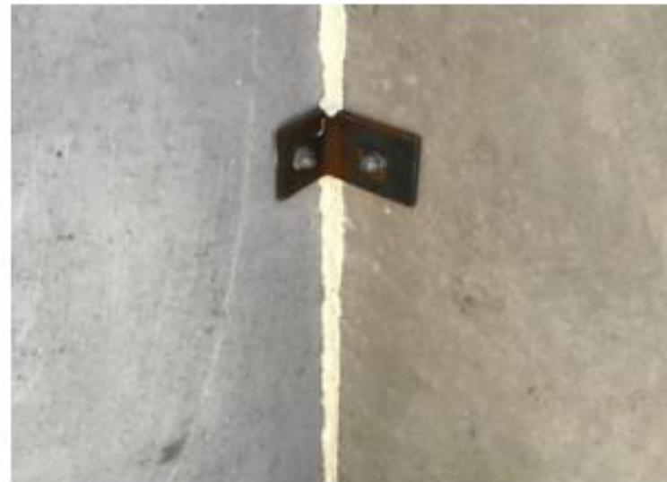
STEP 3: TRIM SPRAY FOAM FLUSH WITH WALL
