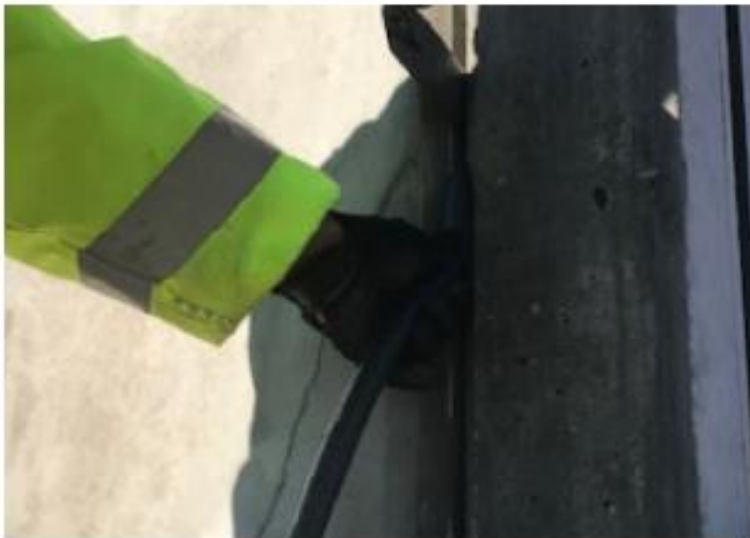
STEP 1: INSTALL BACKER ROD IN JOINT
