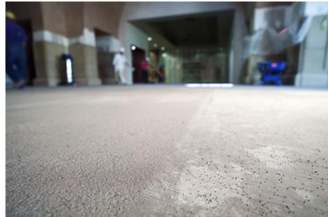
Surface Profile: Shot-Blast Floor Before & After
