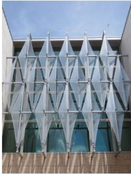
Single Layer ETFE Aluminum Support Structure
