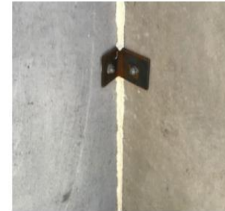
STEP 3: TRIM SPRAY FOAM FLUSH WITH WALL
