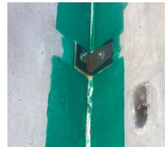
STEP 4: APPLY TRANSITION PRIMER TO BOTH SIDES OF JOINT
