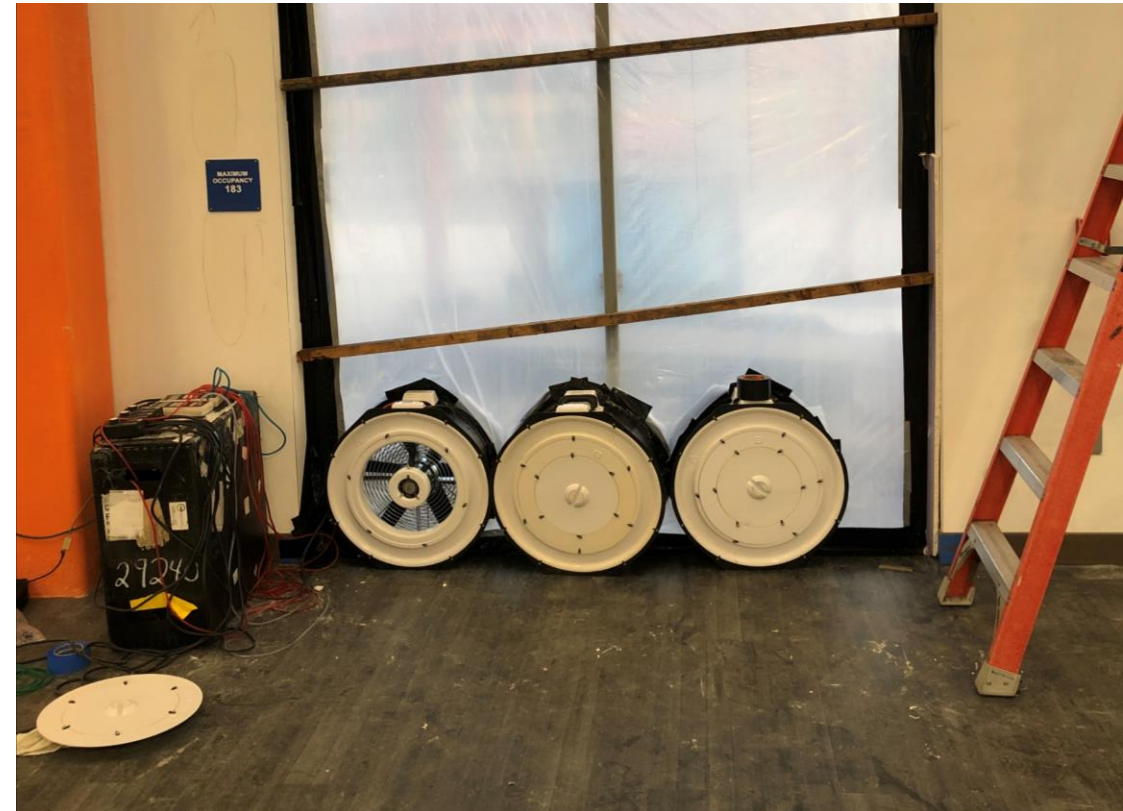
ASTM E779 “Air Leakage Testing by Fan Pressurization”
