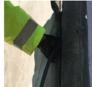
STEP 1: INSTALL BACKER ROD IN JOINT
