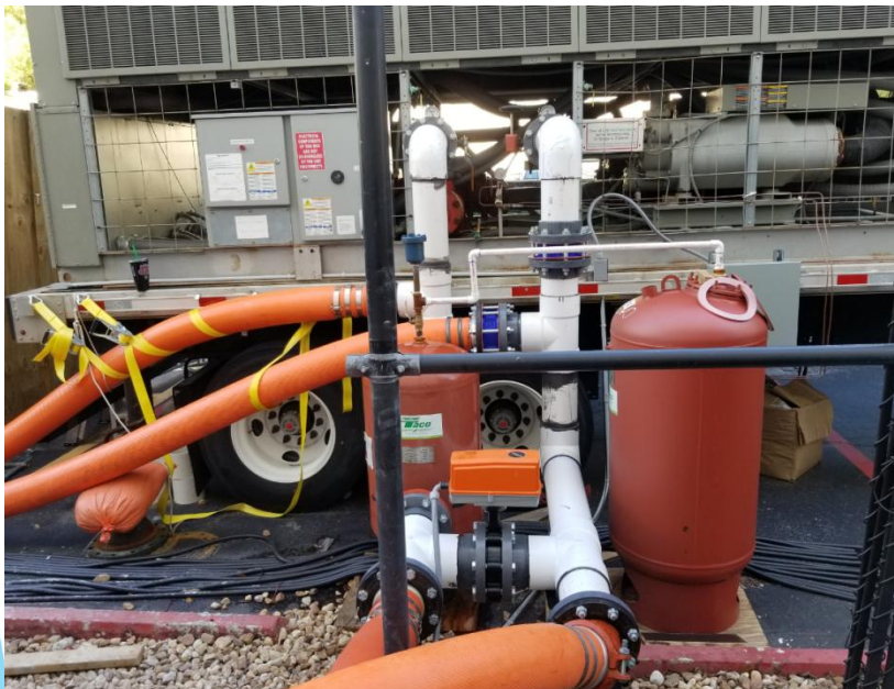
MECHANICAL PARTIAL PLAN- TEMPORARY AIR COOLED CHILLERS LOCATION DURING STAGE 2 OF CONSTRUCTION PHASE TIME OF DURATION: APPROXIMATELY 2 WEEKS
