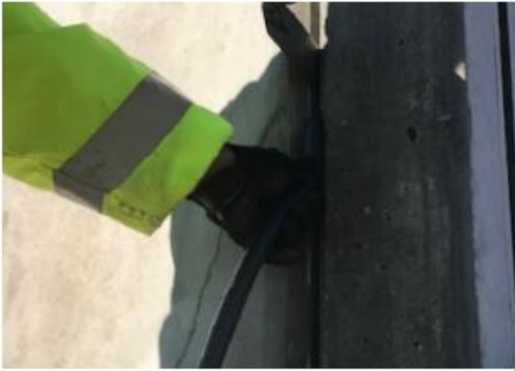
STEP 1: INSTALL BACKER ROD IN JOINT
