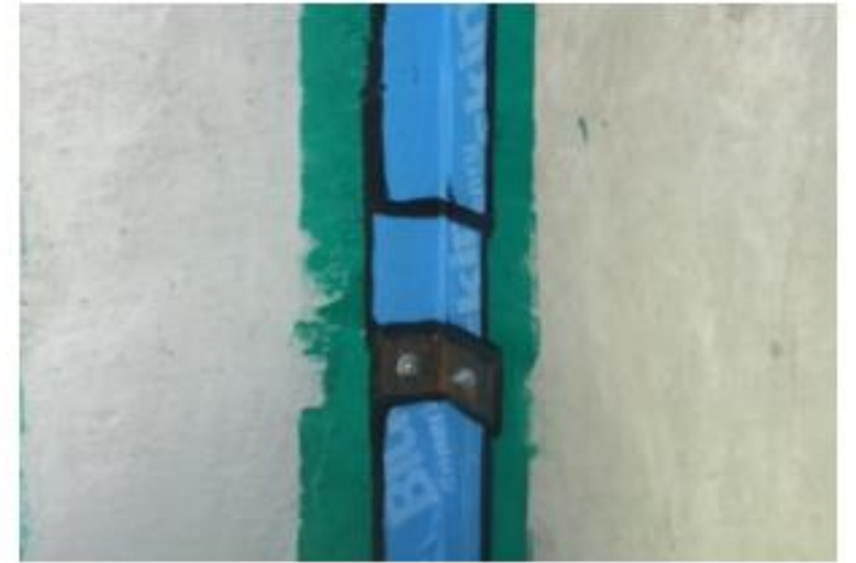
STEP 6: SEAL EDGES OF MEMBRANE WITH BUTYL SEALANT
