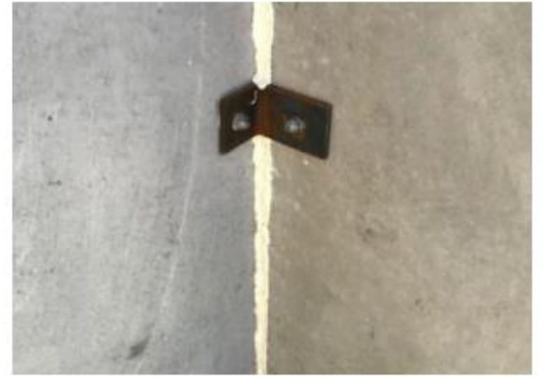
STEP 3: TRIM SPRAY FOAM FLUSH WITH WALL
