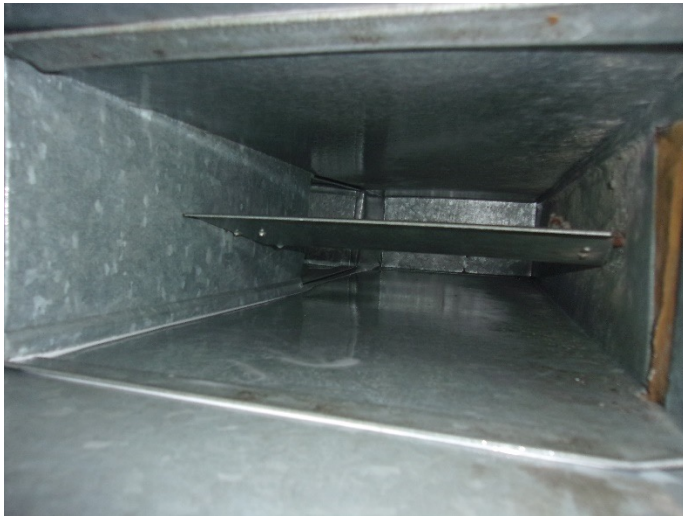
Ductwork - After Remediation
