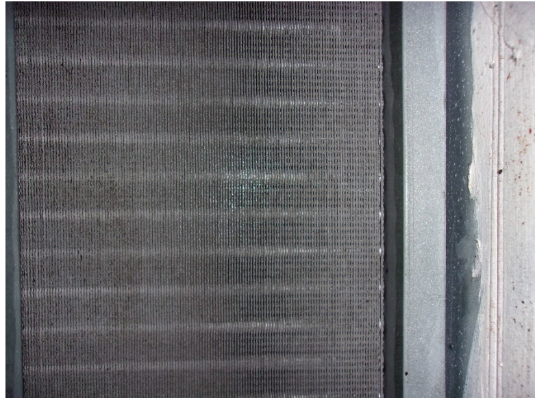
Reheat Coil - After Remediation
