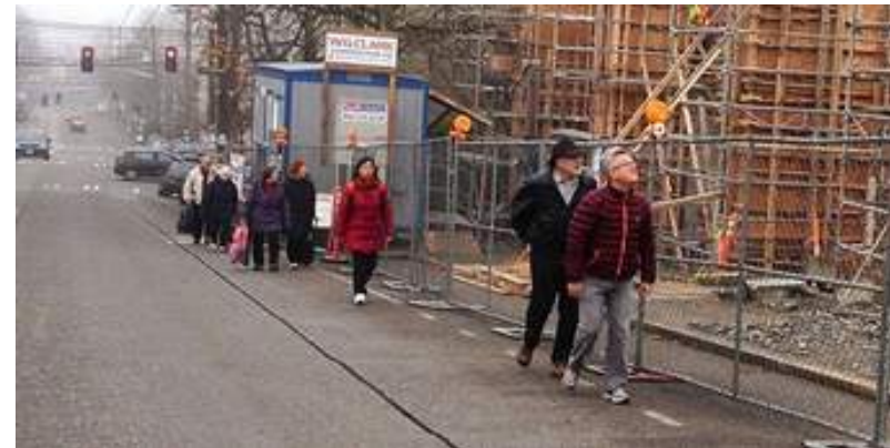
Spillane JP, Flood M, Oyedele LO, von Meding JK and Konanahalli A (2013) Urban high-density construction sites and their surrounding community: issues encountered and strategies adopted by contractors In: Smith, S.D and Ahiaga-Dagbui D.D (Eds) Procs 29 th Annual ARCOM Conference
